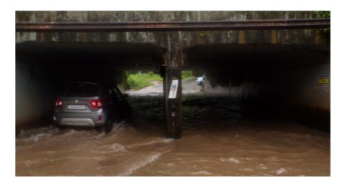
Fig.A.4.4 Inundation in Comba subway during rainfall
